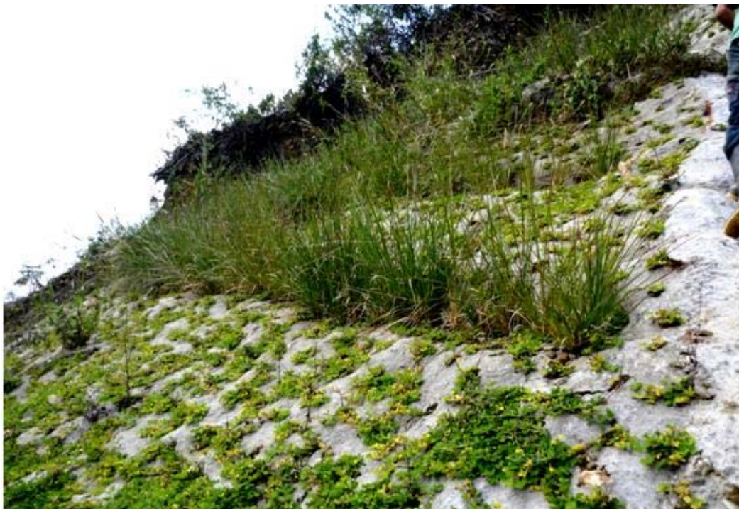
Ecological Mortar- Vetiver- Creeping Forage Peanut (Arachis pintoi) Mountain Highway "Las Palmas" Km1+500 - Medellin. Antioquia
