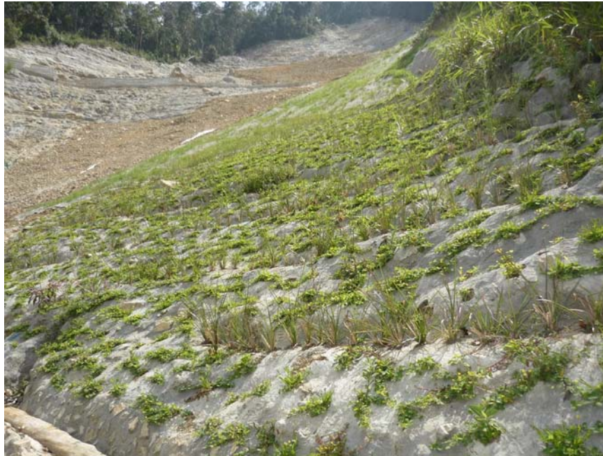
Ecological Mortar- Vetiver- Creeping Forage Peanut ( Arachis pintoi ) Mountain Highway "Las Palmas" Km1+500 - Medellin. Antioquia
