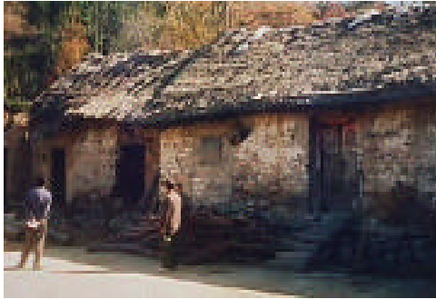
Housing condition in Changpu Township
