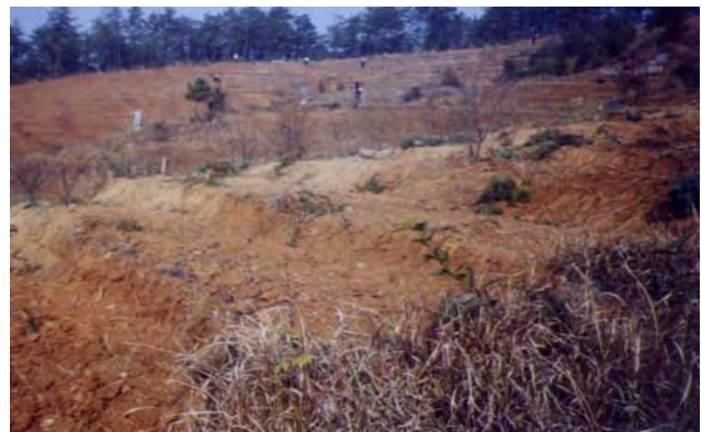
Terraces in construction
