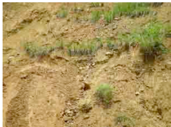
Young vetiver stopped slope slides (soil below the vetiver hedge was slide)
