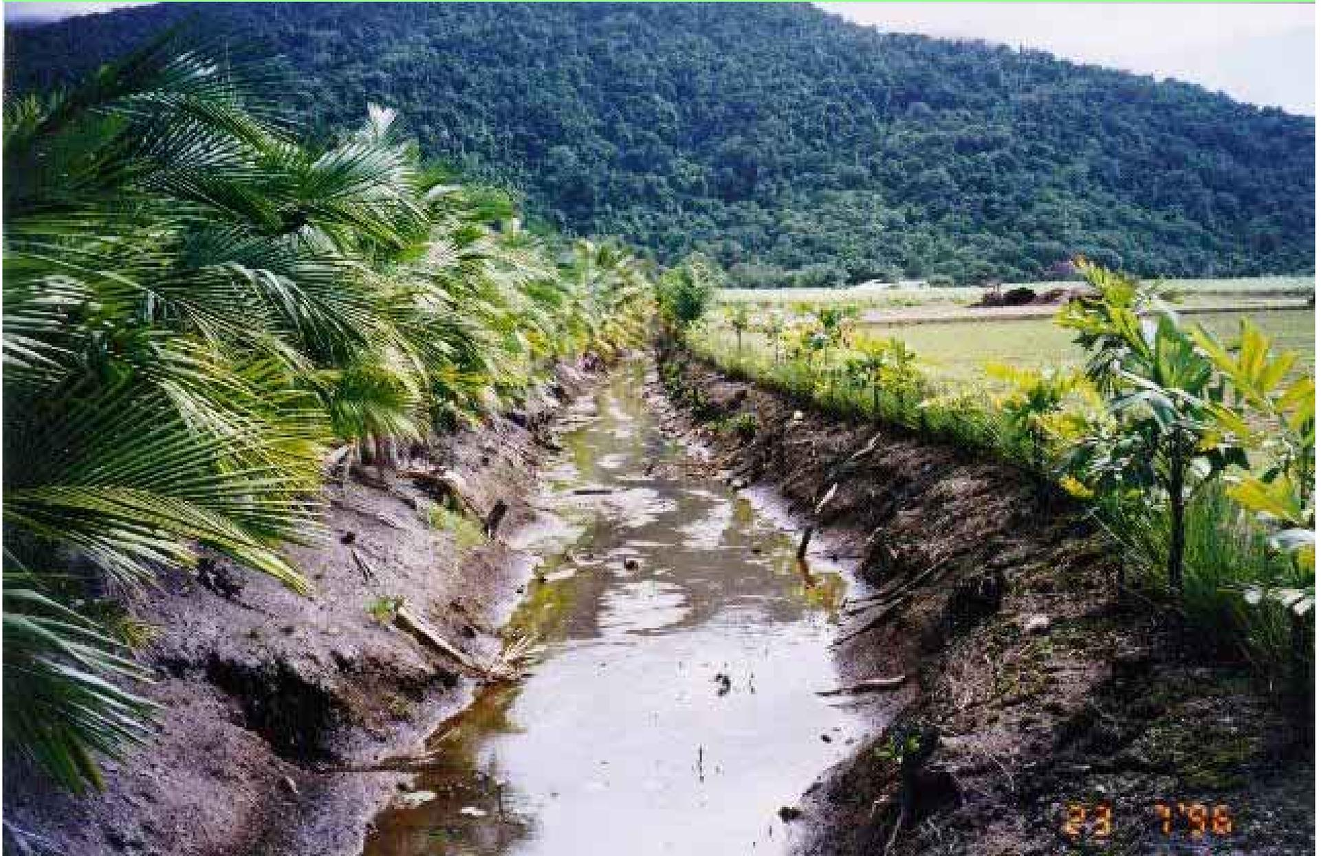
Typical erosion on the bank of a drain on acid sulphate soil
